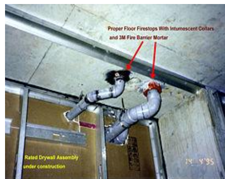
Nortown Castles, North York (now Toronto), Ontario, Canada, April 1995. Set-up for subsequent code infraction in plastic pipe wall penetrations. Improper hole sizing. Firestops (in the walls) the plumber considered to be the drywaller's responsibility. Floor openings are properly done in this case, with intumescent pipe collars and firestop mortar. The intumescent will expand and choke off the melting pipes. Drywall mud does not work as a plastic pipe firestop in the wall.
